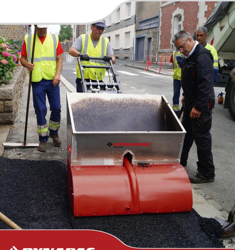
**THE DYNAPAC COMPACT EQUIPMENT RANGE** compliments our larger compaction & paving equipment to get the job done in relatively confined spaces. Dynapac S100 is a self-propelled mix spreader best suited for use in relatively small and tight spaces. It helps you deliver consistent results by allowing precise height and material flow adjustment. You will experience a new level of operating comfort thanks to the swivel castor wheels and all the controls that are located at the fingertip.
